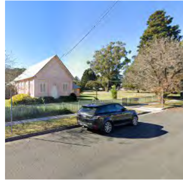
D32 Mittagong Uniting Church Hall
