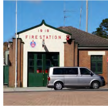
D50 Mittagong RFS Comms Centre
