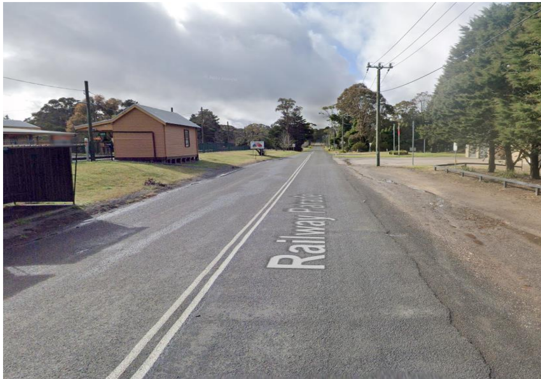
Image 3 – Pre-construction image of the subject location (looking east)
