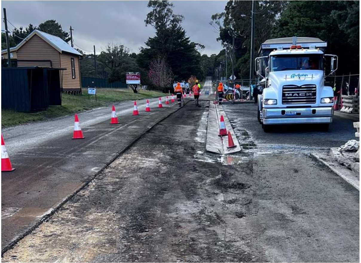
Image 4 – Civil works during construction showing the dish drain (looking east)
