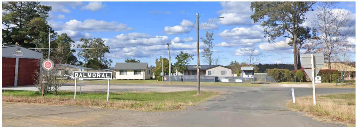
Image 4 – Existing north level crossing between Railway Parade and Wilson Drive, Balmoral Village (looking east)
