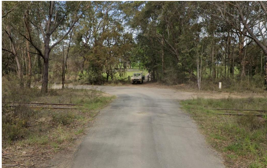
Image 6 - Existing south level crossing between Railway Parade and Wilson Drive (looking east)
