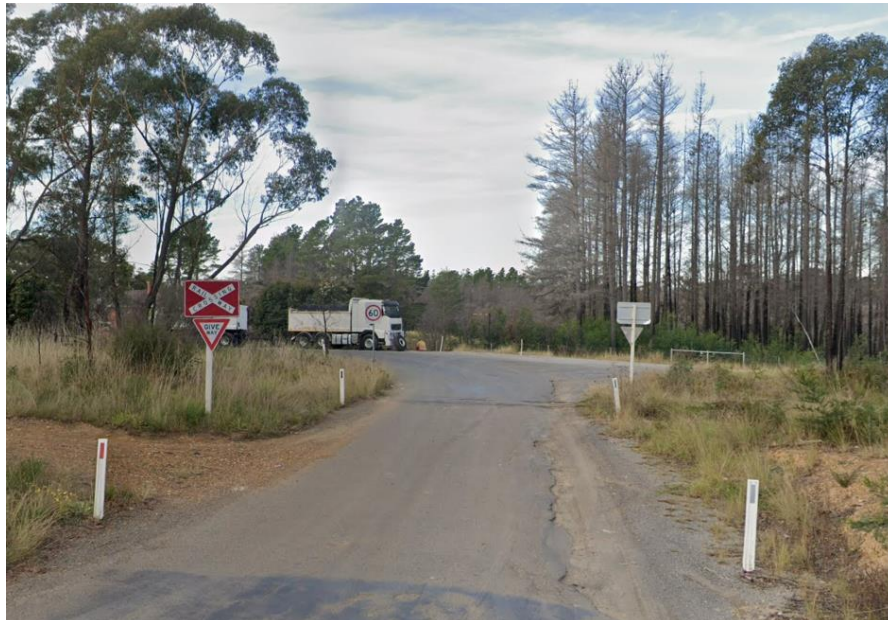
Image 2 – Existing level crossing between Wilson Drive and East Parade, Buxton (looking east)
