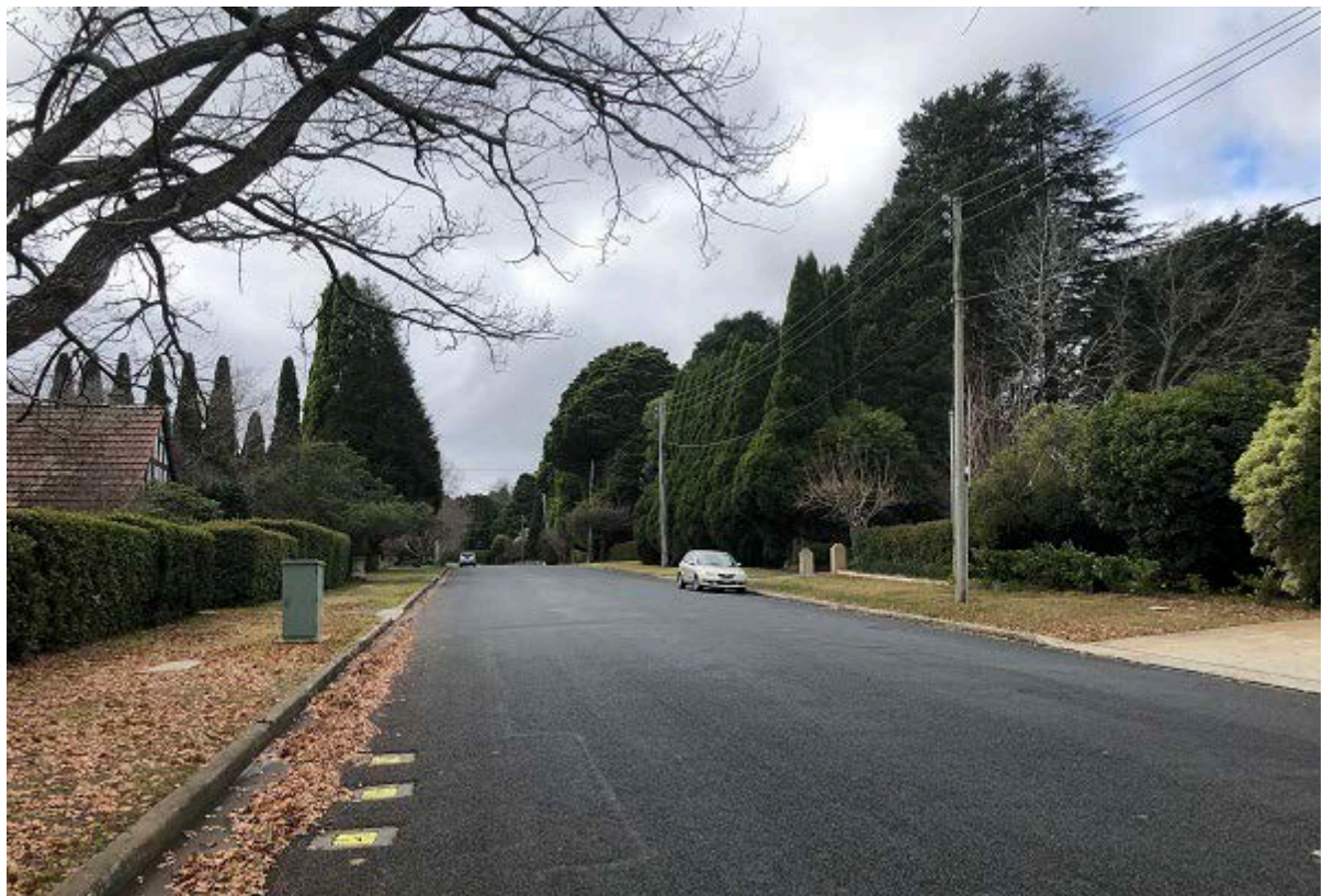
Figure 6—Aitken Road from Kangaloon Road looking north
