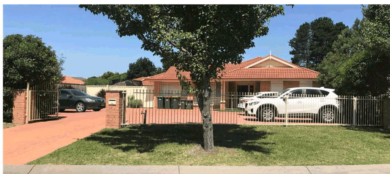
Figure 3: Site as viewed from the south west showing car parking and hard stand areas within the front setback
