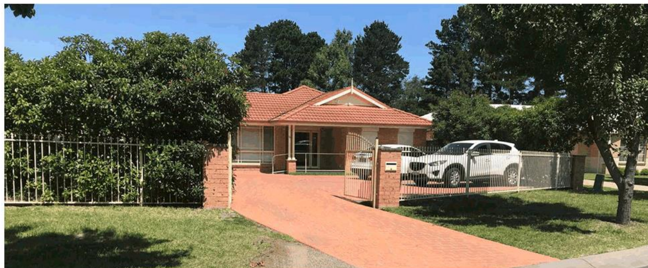
(Attachment 2) Figure 2: Site as viewed from the north west showing accessible entry porch and doorway
