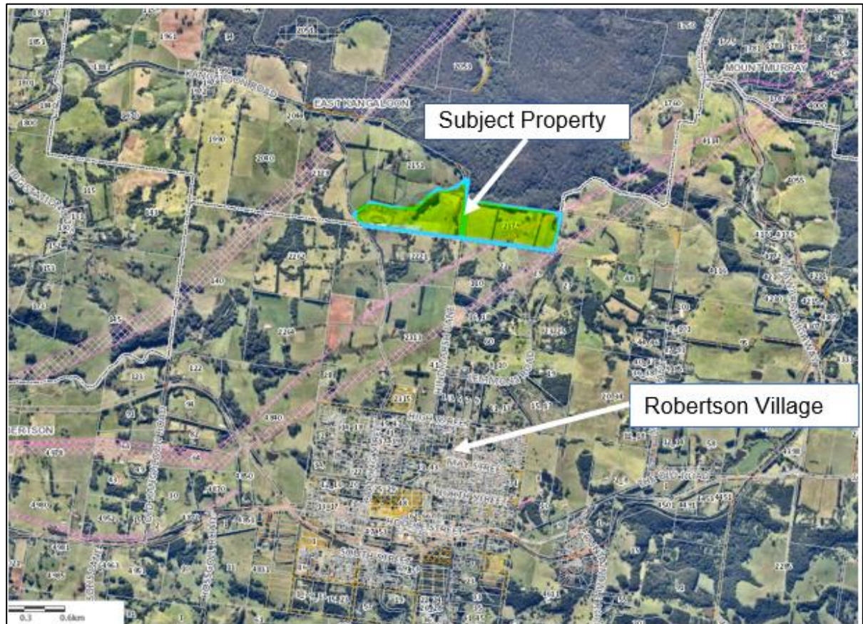
Figure 3: Aerial Image and locational details marked (site and Robertson village)
