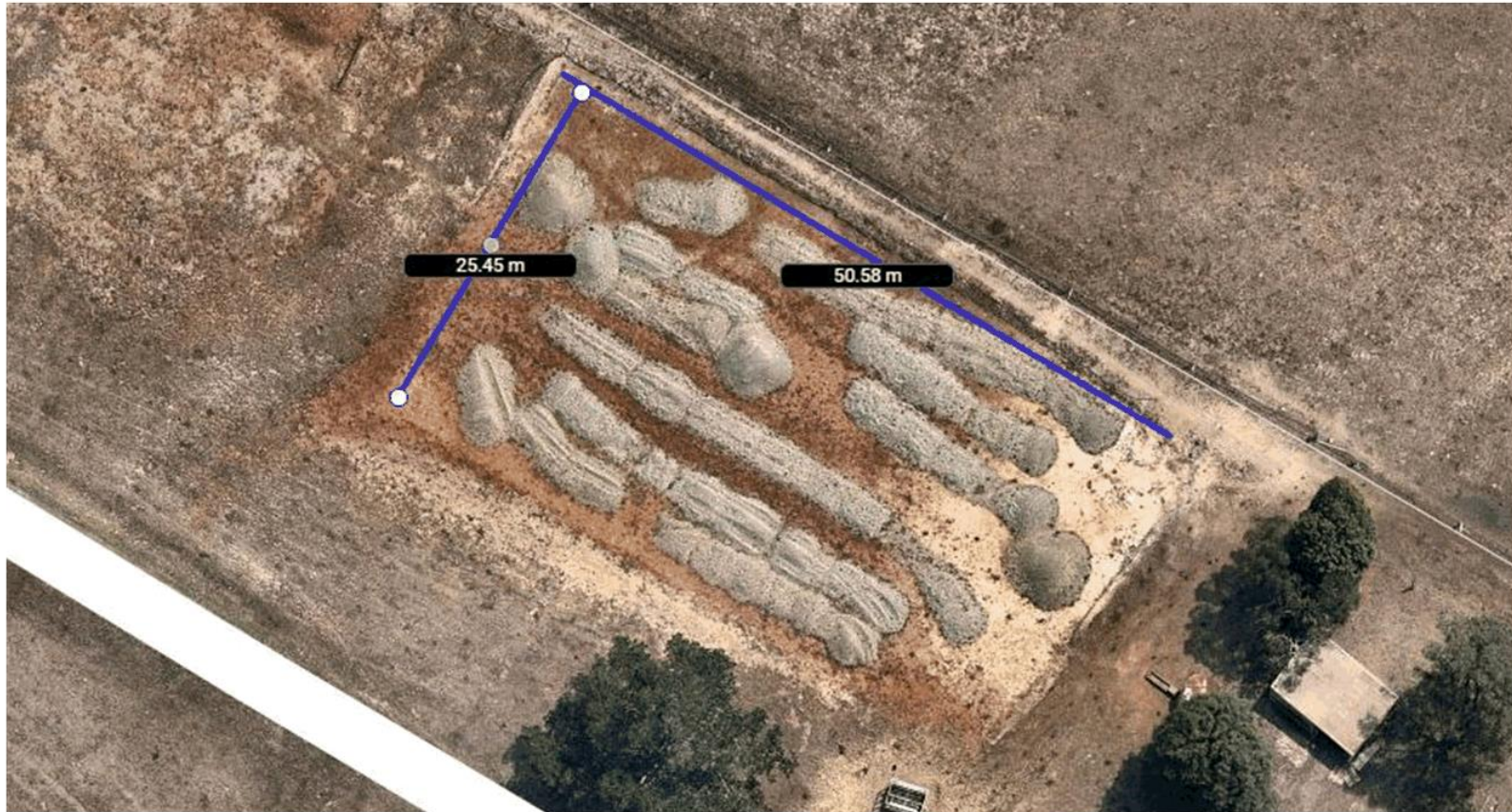
Image 3 – Excavation Footprint – 30 January 2020
