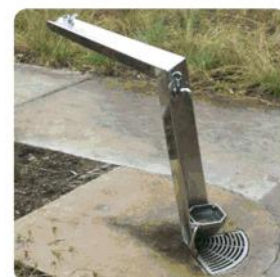
New drinking fountain
