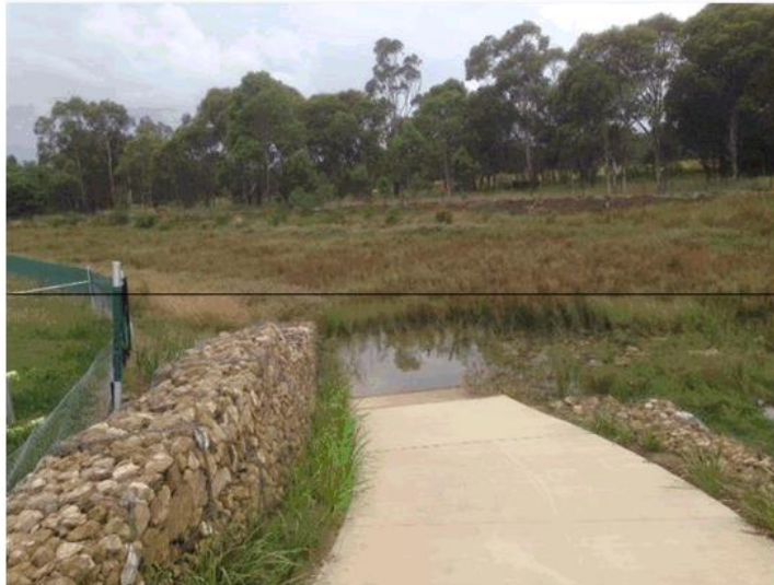
Example of a Bio-retention System at Renwick
