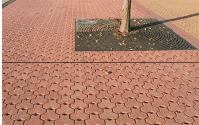
Example of Porous Pavement
