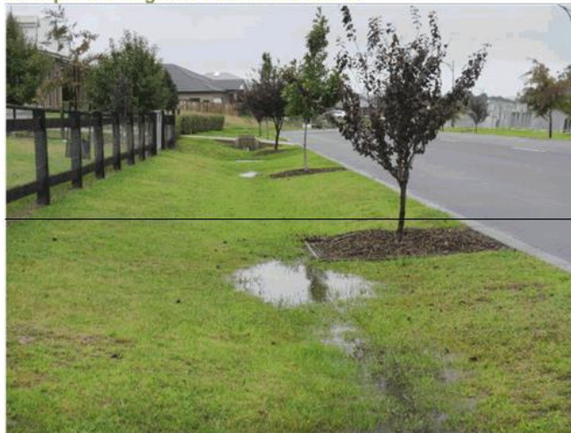
Example of a Grass Swale at Renwick
