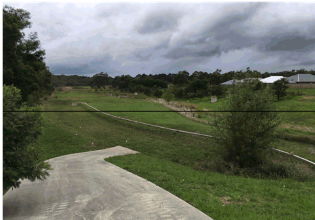
Example of an Infiltration System at Renwick
