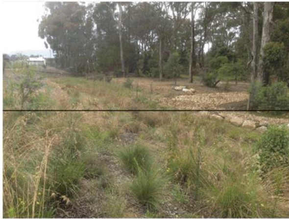
Example of a Vegetated Swale at Renwick
