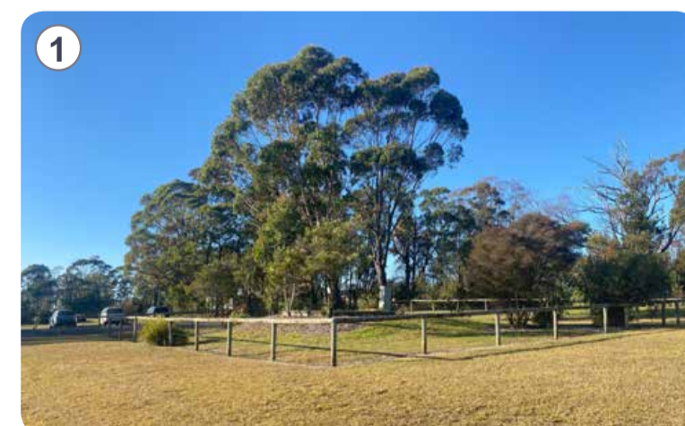
Septic Tank & Existing fencing
