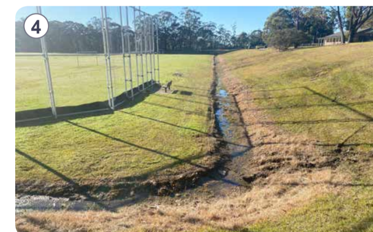
Existing trench drain/swale
