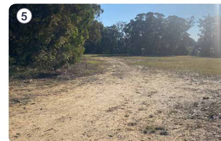
Eroded driveway entry to pony club
