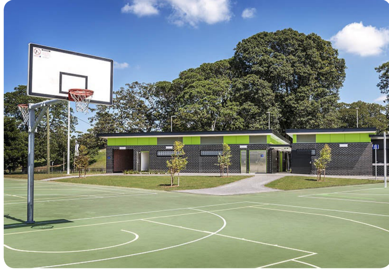
Half-court basketball with linemarking
