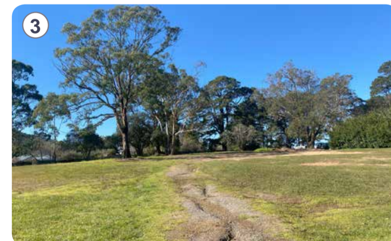
Open turf area with evidence of drainage runoff
