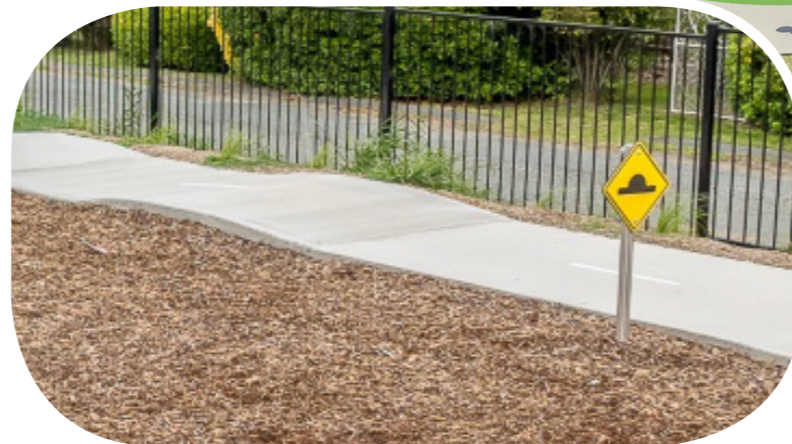
Line marking with bumps in the path added to scope.
