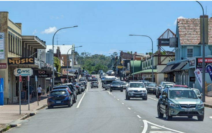
Bong Bong Street has a 20m wide road reserve containing two travel lanes, parallel parking lanes and a footpath either side.
