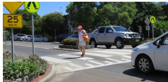
Raised pedestrian crossing, Kiama NSW
