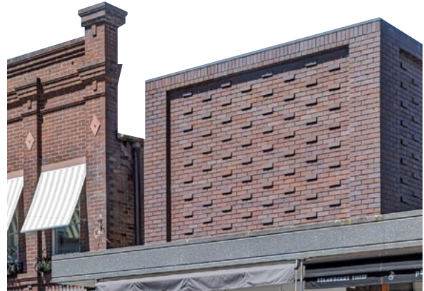
Bowral Blue bricks are a unique local material and contribute to the town centre's character and identity. Here are examples of heritage and modern use.
