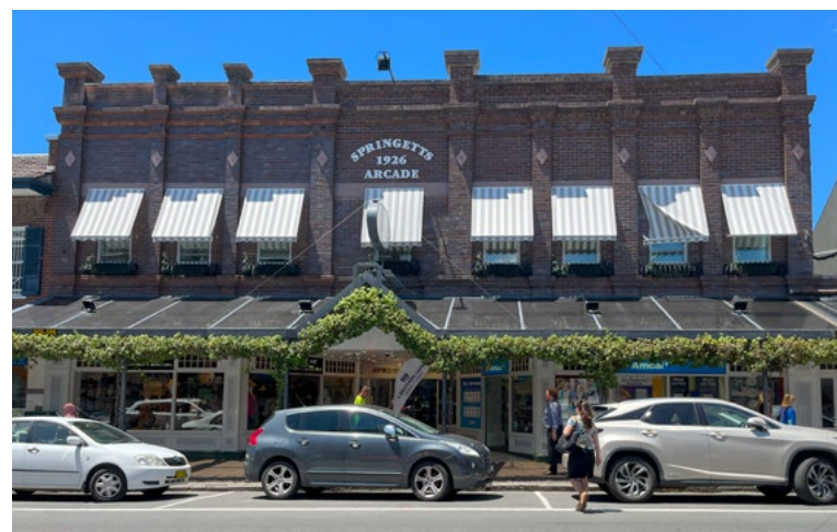
Springett's Arcade character building on Bong Bong Street
