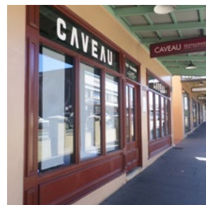
Retention of original shopfront elements where possible
