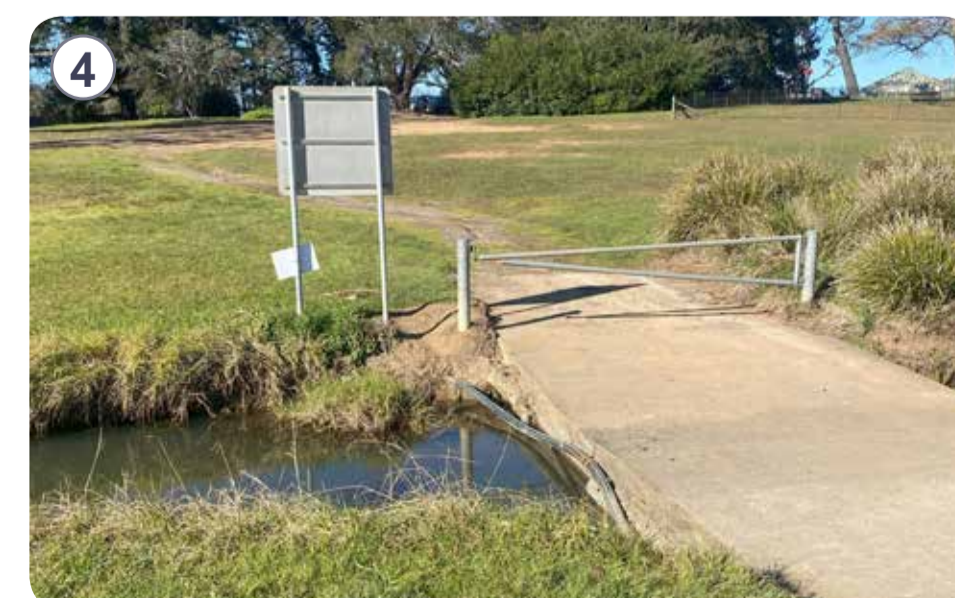
Existing maintenance vehicle bridge & pedestrian access
