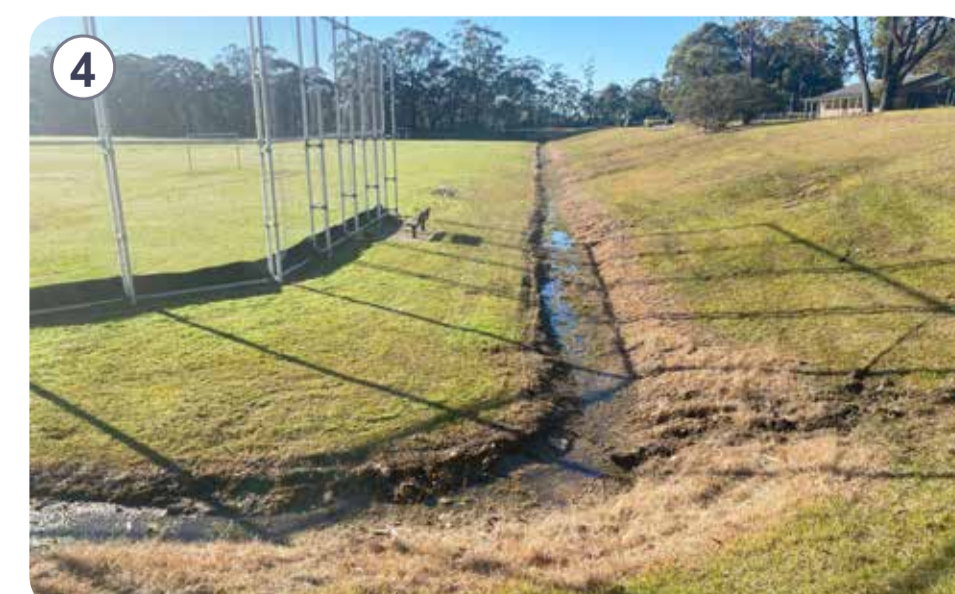
4 Existing trench drain/swale
