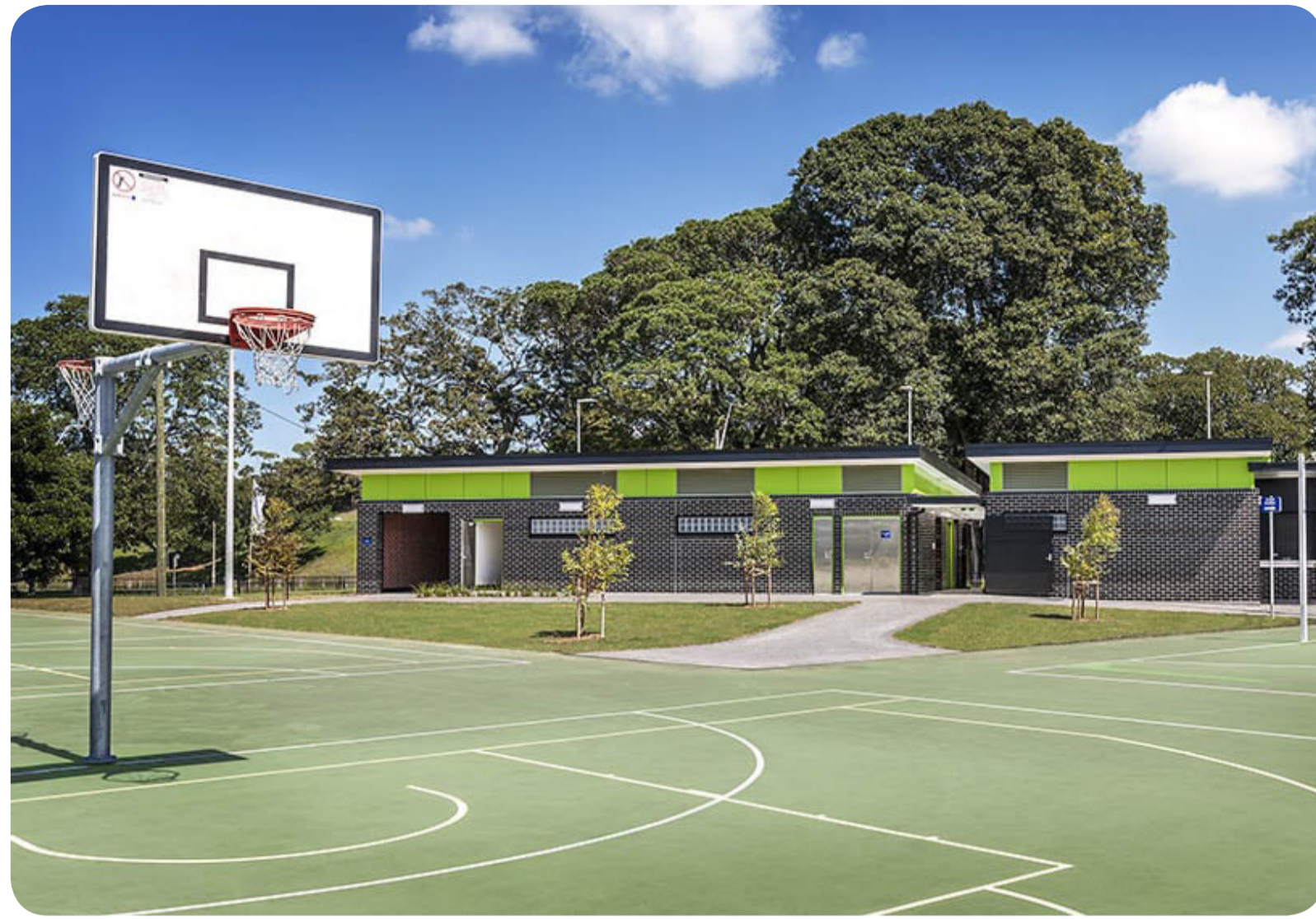
Half-court basketball with linemarking
