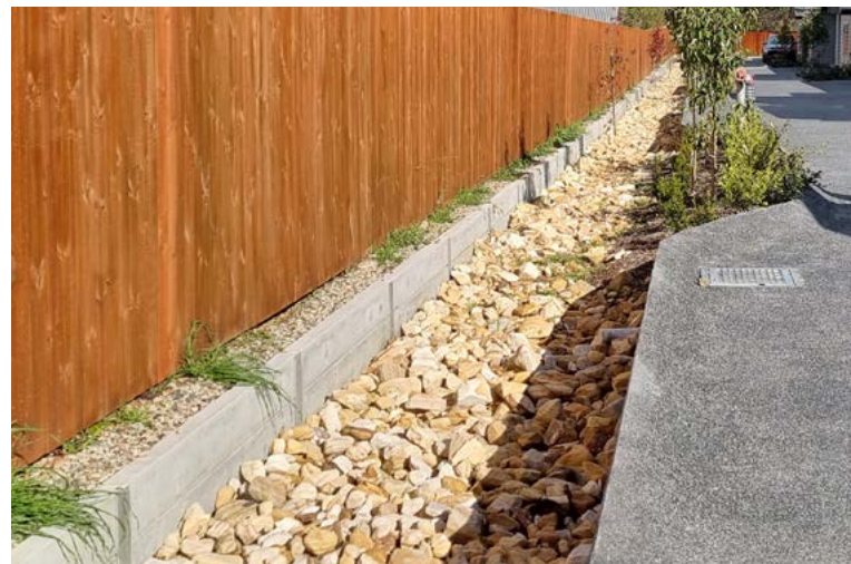
Figure 58 Stormwater management should be considered as functionally and visually integrated into the overall design
