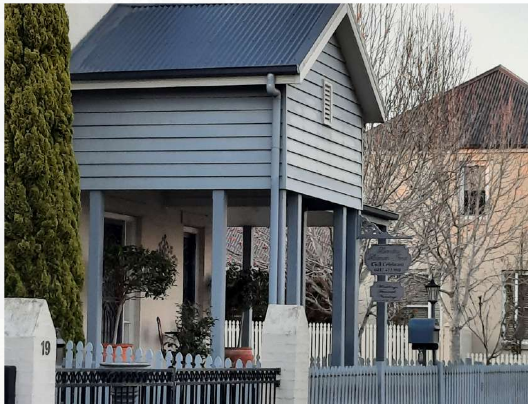
Example of a home business in Tullimbar, NSW
