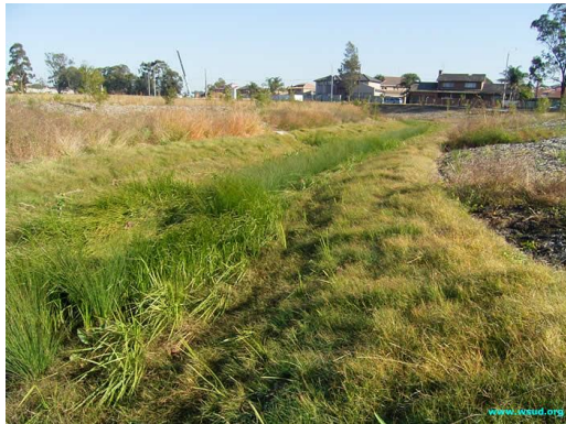
Photo*: Vegetated swale, Fairfield New South Wales
