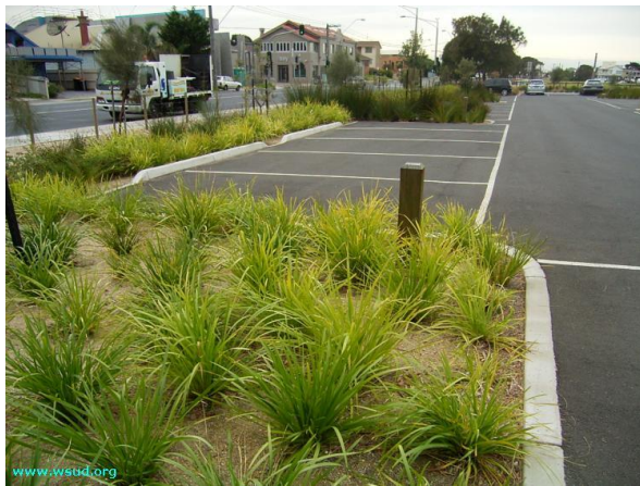
Photo*: Example of rain garden (bioretention basin) adjacent to car parking bay at Beachside Car park (Melbourne), Victoria.
