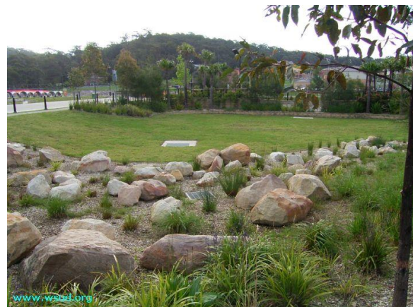
Photo*: Onsite retention basin and vegetated filter integrated into the surrounding landscape, Warriewood (Pittwater Council), Sydney.
