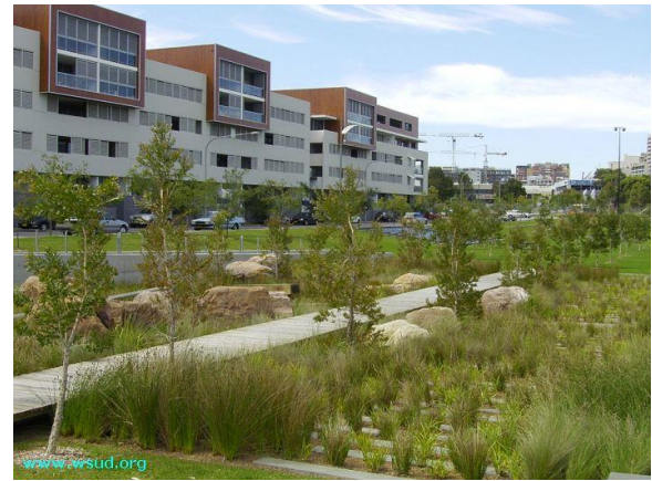
Photo*: Bioretention basin, Victoria Park, Sydney.
