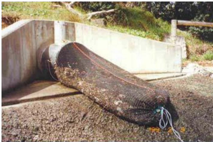
Photo: Gross pollutant trap at Umina, Gosford City Council, New South Wales (Source: www.gosford.nsw.gov.au ).
