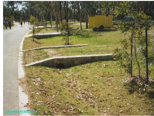
Photo*: Grassed swale with adjacent driveways, Cairnlea, Brisbane Queensland.
