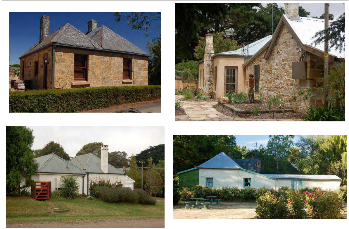
Figure A8.13—Successful additions retain the original cottage roof form
