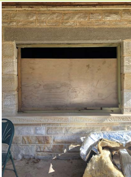
After project photo: showing reinstated original window layout with sill
