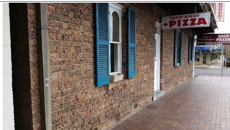
Before project photo: Photo courtesy D. Keen
