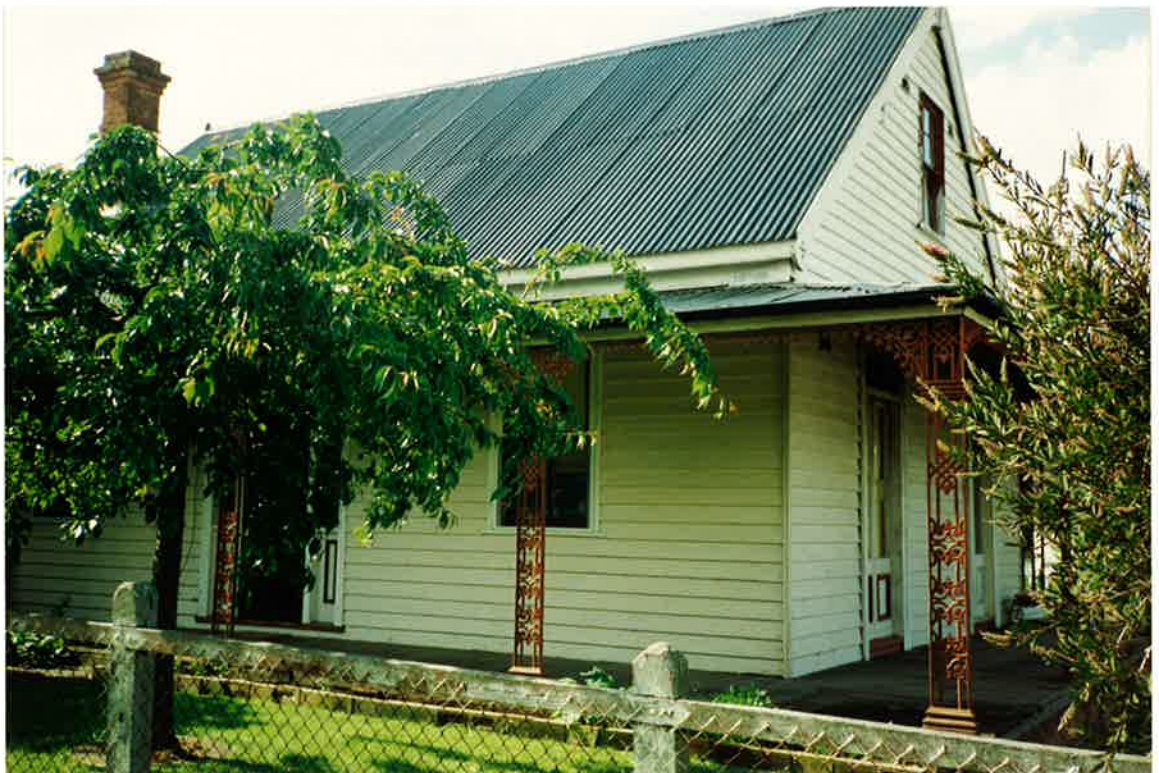
PLATE 55: New Sheffield residences with cast iron verandah columns
