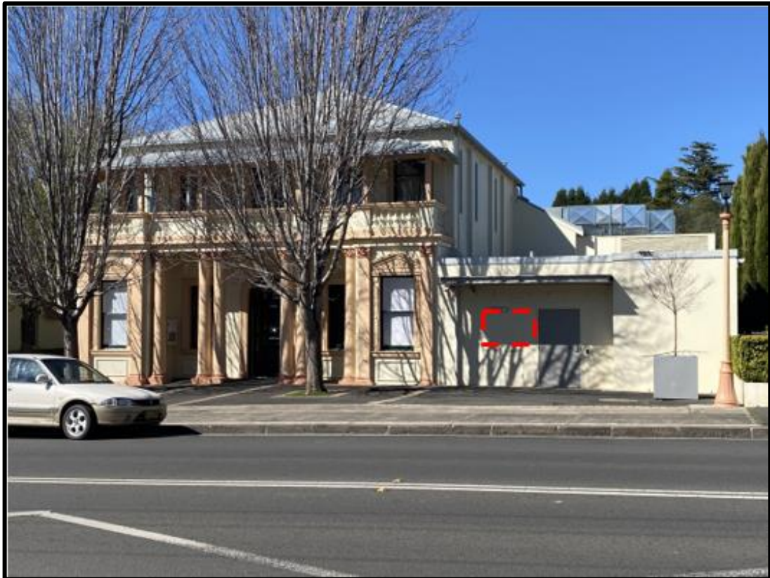
Photo of front of Bowral Memorial Hall (western side, facing Bendooley St), with the location of the sign on a recent extension to the Hall, outlined in red.
