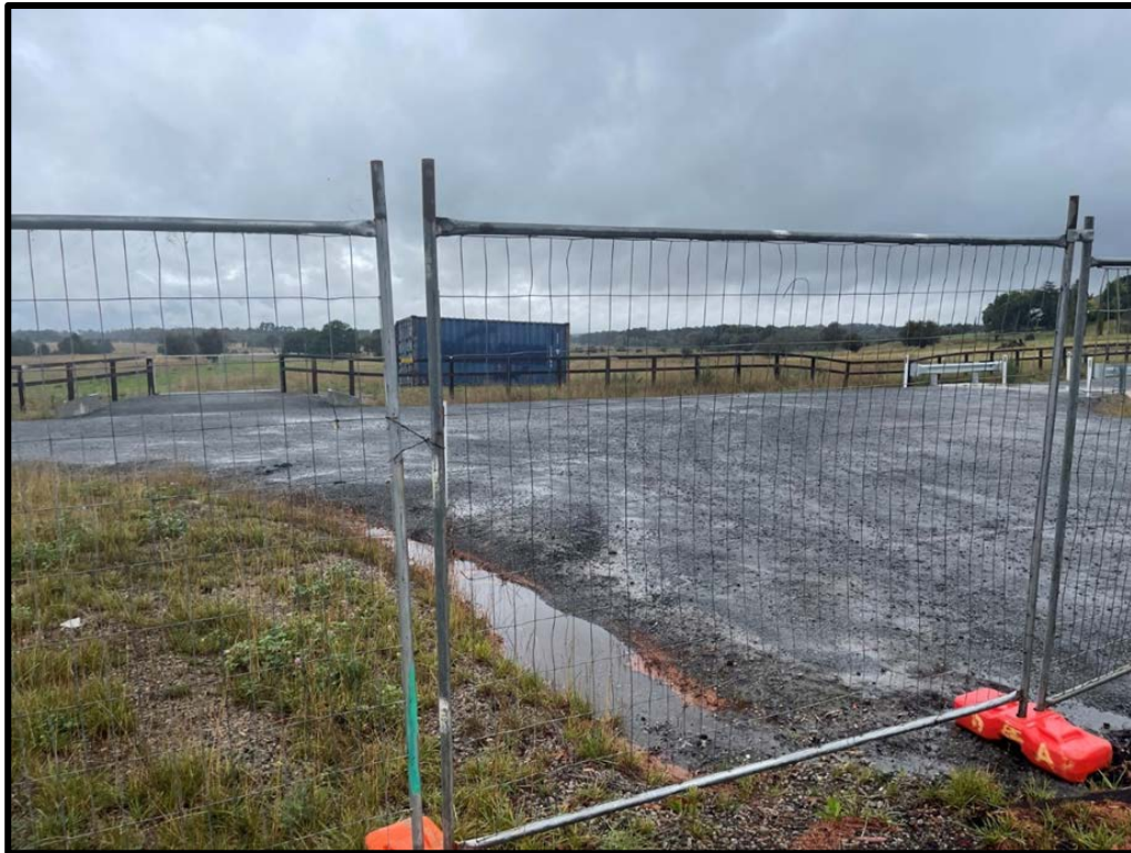
Figure 3: Subject site viewed from Moss Vale Road (south-east orientation)
