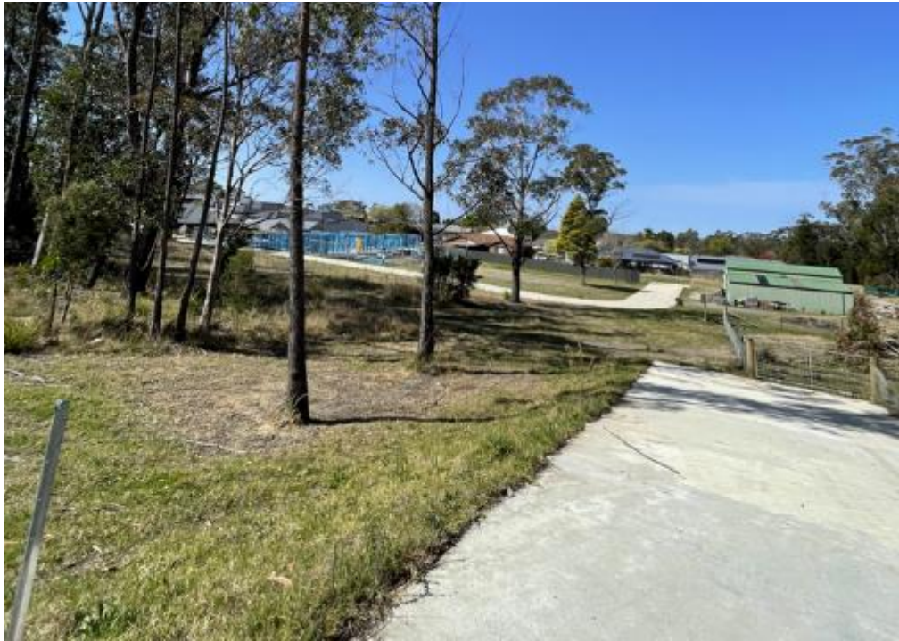
Figure 3: Existing driveway as viewed from Cordeaux Street. Source: CPS Site inspection 13 September 2023
