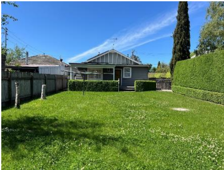
Figure 4: Eastern elevation of the dwelling as viewed from the rear yard.
