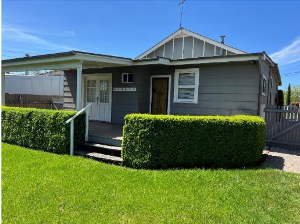
Figure 7: Facing east towards the minor demolition of existing rear deck to accommodate the proposed kitchen, setting and dining extension. Source: CPS site inspection, 17.10.2024.
