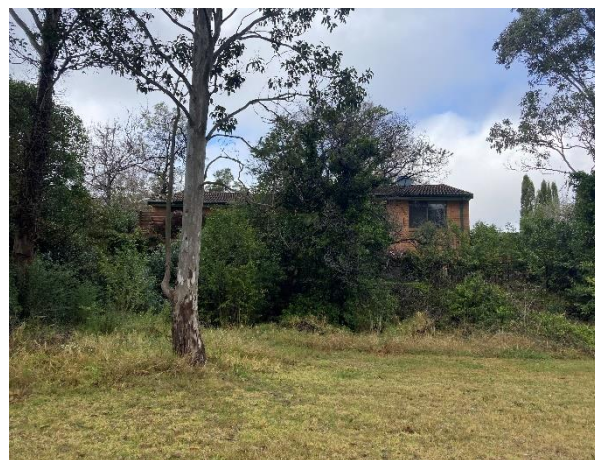
Figure 8. The rear adjoining neighbours (3 dwellings) at 6 Holmhale Street, which will be
