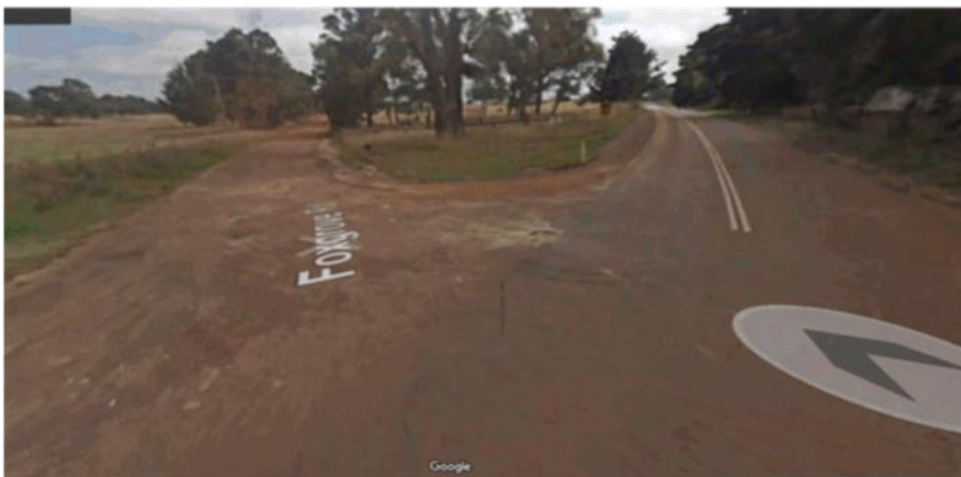
Figure 3 – Existing Intersection of Foxgrove Road / Canyonleigh Road
