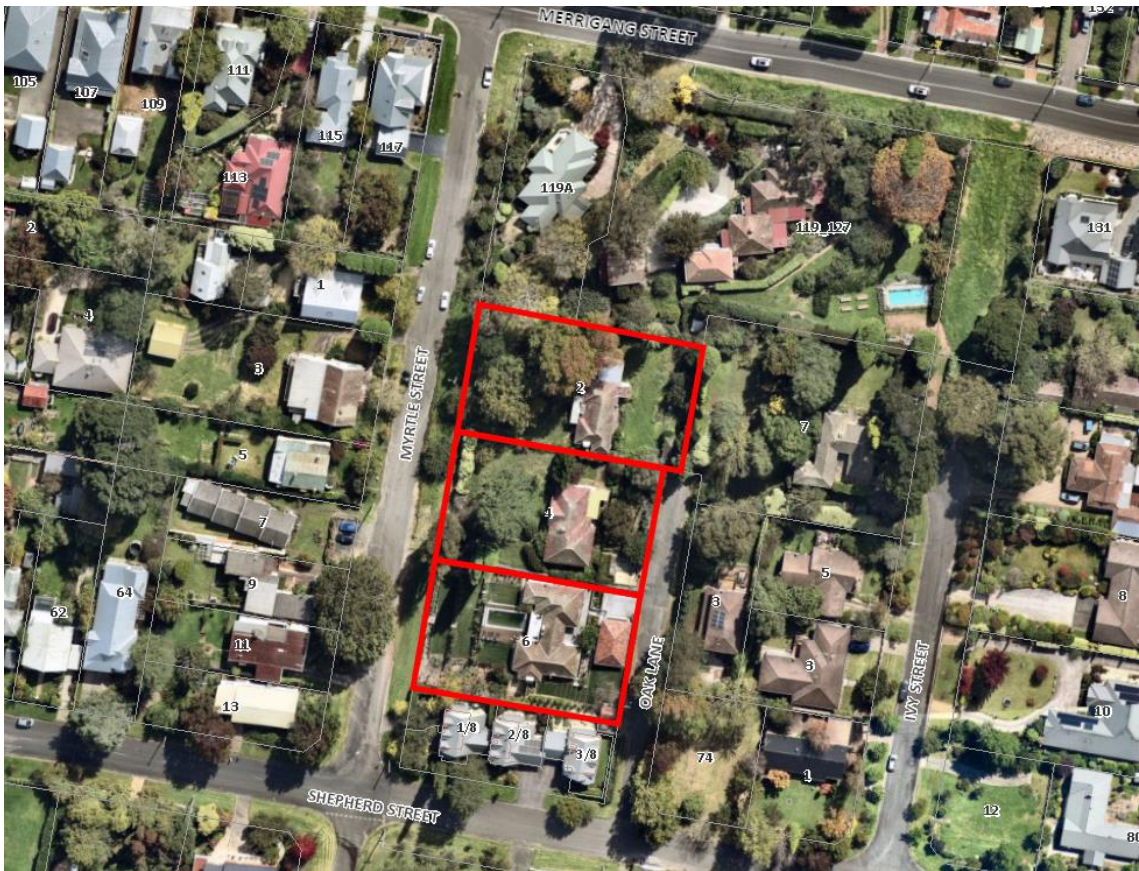
Figure 1: 2, 4 and 6 Myrtle Street, Bowral (outlined) in the context of the surrounding area (Source: Nearthmap, 16 April 2022)
