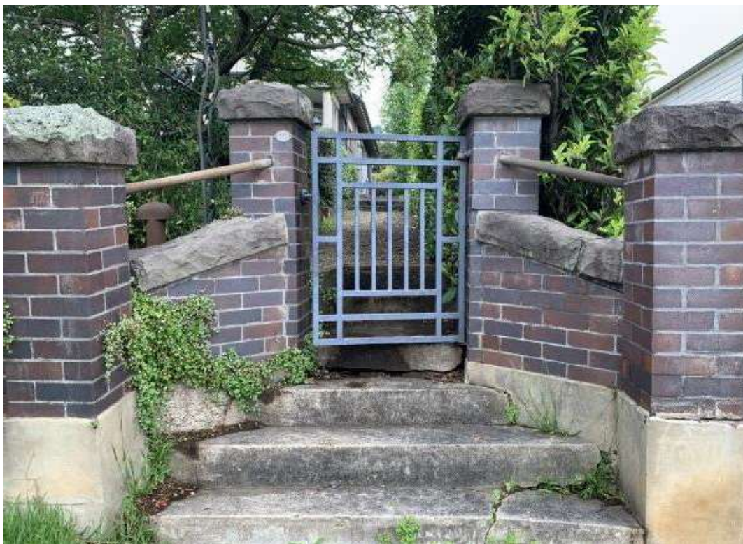
Figure 13: Detail of entry gate with aesthetically significant brick and trachyte fence (2022).
