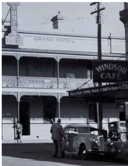
Figure 2.11 From 1924 the refreshment rooms were known as the Windsor Cafe. This photograph of 1949 depicted the signage of the cafe mounted on the new cantilever awning
