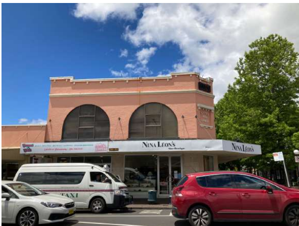
Figure 7.2 Styros Corner (1922) opposite the subject site with a splayed corner, parapet and arches to the upper level
