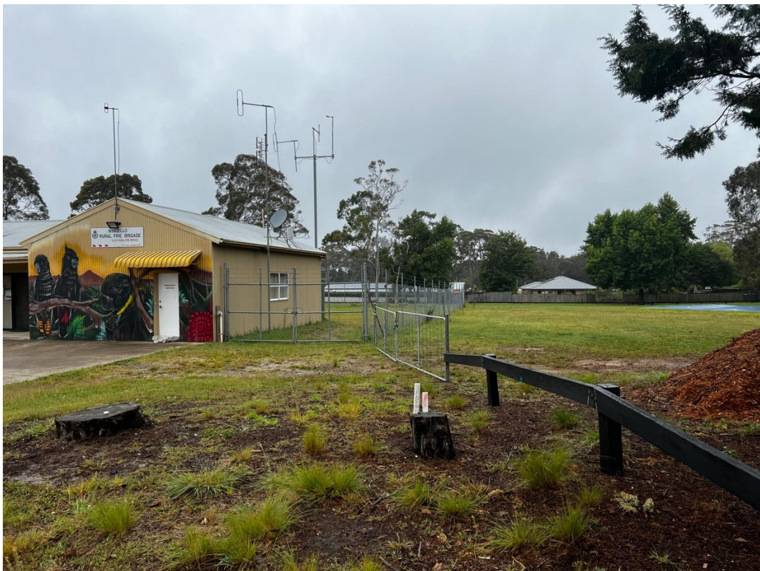
Figure 15: Rural Fire Brigade shed and boundary fencing separating Casburn Park
