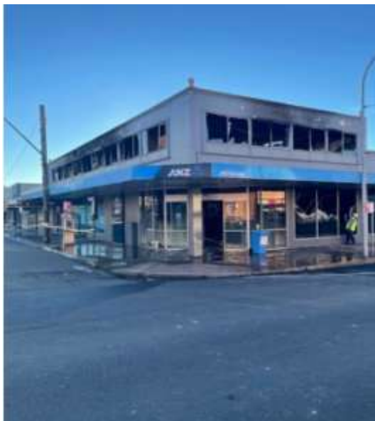
Figure 2.13 The building after the fire in July 2021
