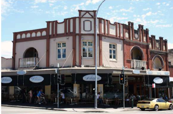
Figure 7.1 Typical Edwardian Federation style shops. Note the higher element and splay to the corner, the use of arches and brick detailing
