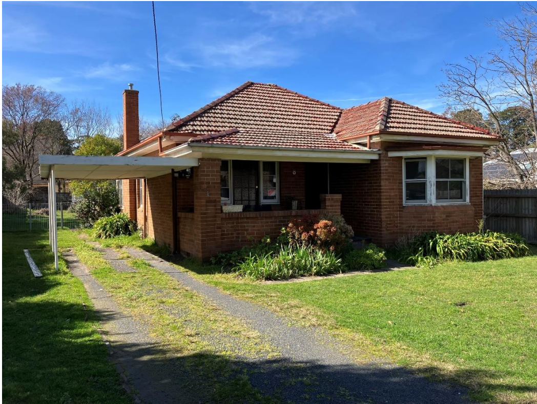
Figure 12: Existing dwelling at No.8 Kangaloon Rd Source: Site inspection, 23 August 2024
