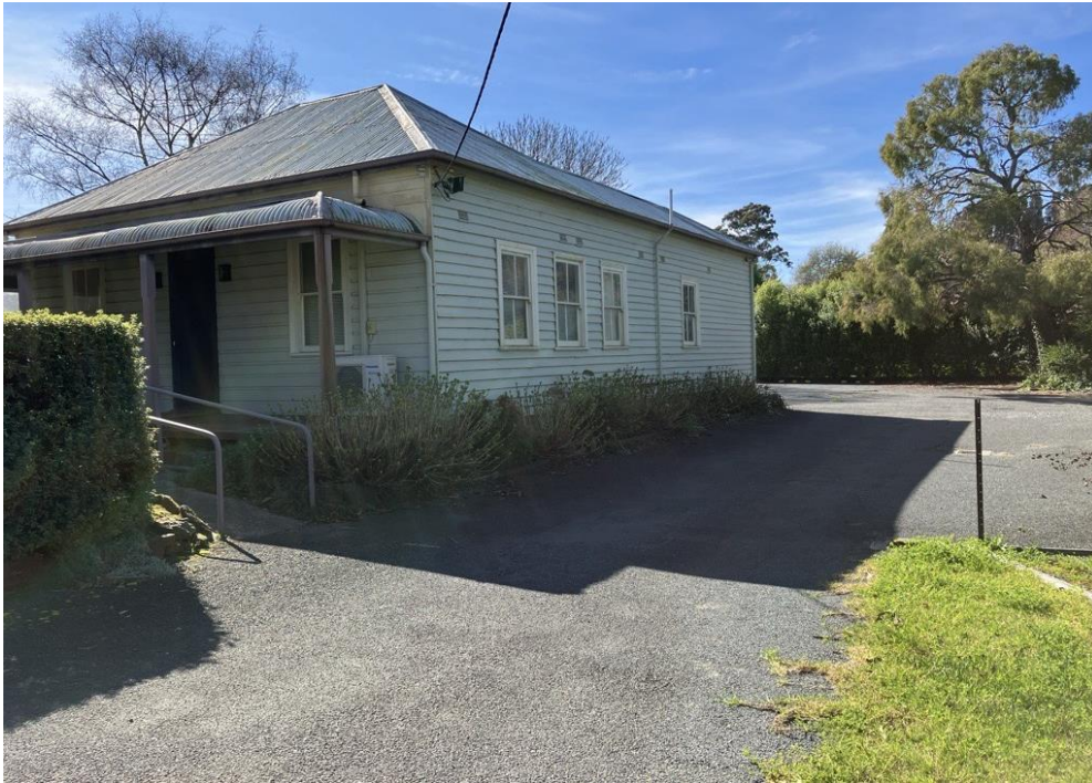
Figure 10: Existing dwelling at No.6 Kangaloon Rd Source: Site inspection, 23 August 2024
