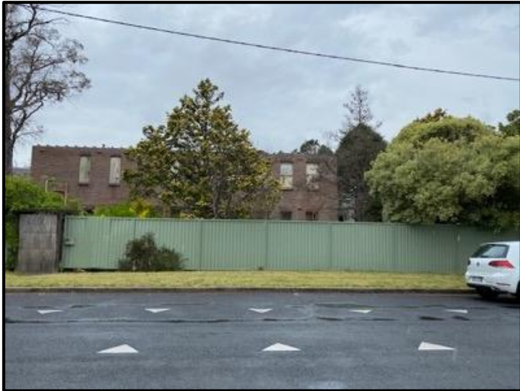
Figure 4: Photo of Northern Elevation from across Alfred Street (Source: Applicant)
