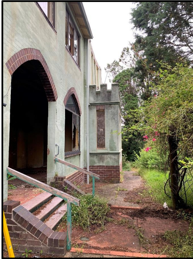
Figure 6: Photo of Existing Building Entrance from Alice Street (Source: Council)
