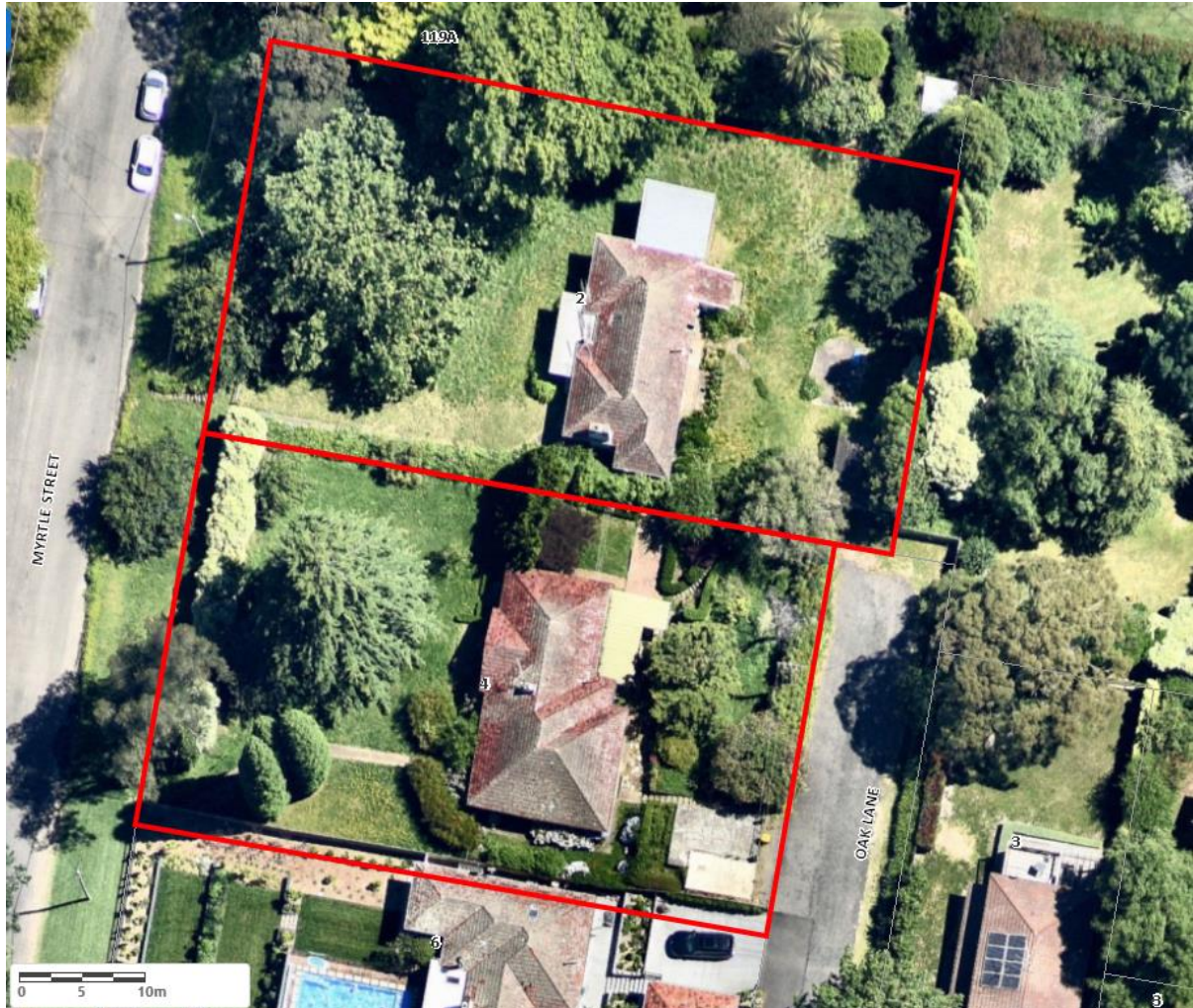
Figure 1: Aerial photo of 2 & 4 Myrtle Street (Source: Nearmap, December 2021).
