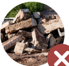
Demolition waste (bricks, fibro, concrete)
