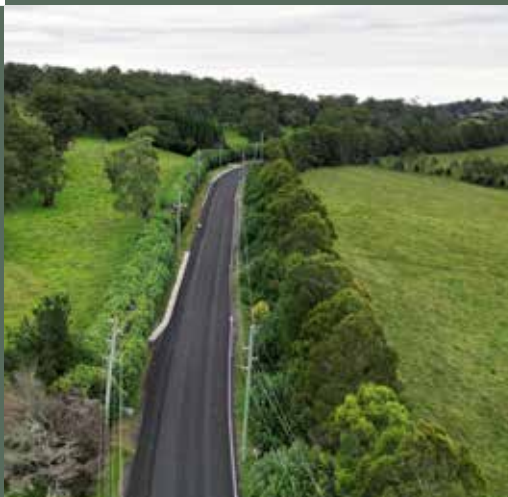
Old South Road rehabilitation project completed
