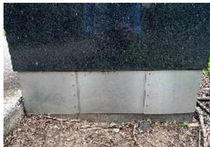
Fig 12: M1 stainless steel skirt at base rivets at rear
