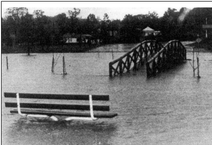
Figure 6. The park at Mittagong Road during 1986 Floods (Bewsher Consulting Pty Ltd, 2009)
