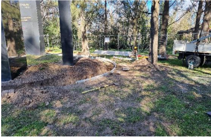
Figure 40. Photo during the modification works 13/07/2023. (McCann, 2023)
