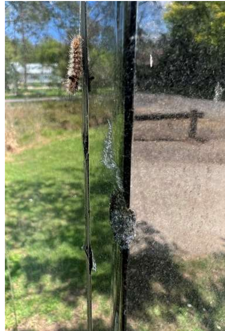
Fig 36: M9 losses to granite on SW edge below cracking on inscription panel
