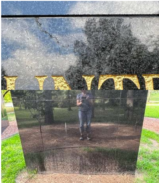
Fig 24: M5 open crack above Country
