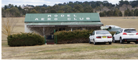
② Main Vehicle Entry, Moss Vale Rd
