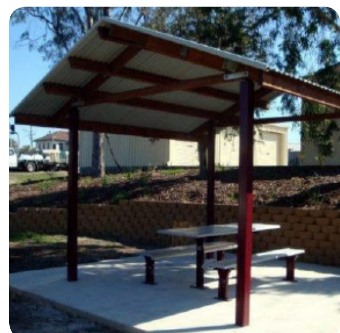
Upgrade existing picnic settings
