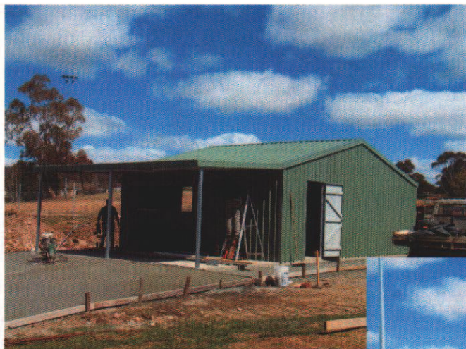
Newly constructed canteen and toilets
