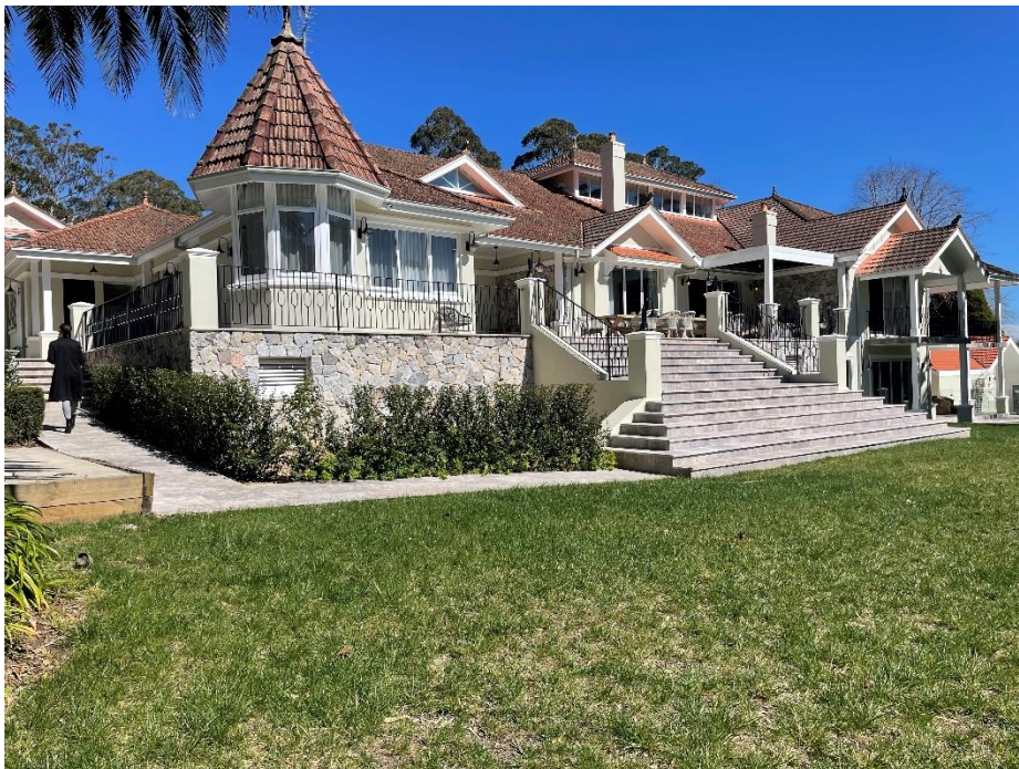
Figure 4: View of Existing House from Northern Boundary. Source: Site inspection 27 August 2024
