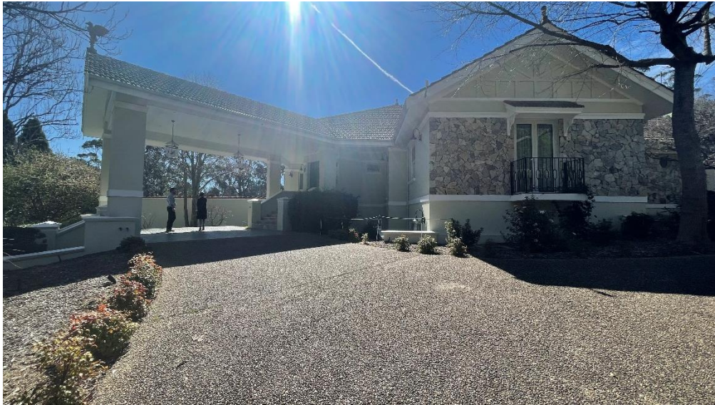
Figure 5: Primary entrance to the building Source: Site inspection 27 August 2024
