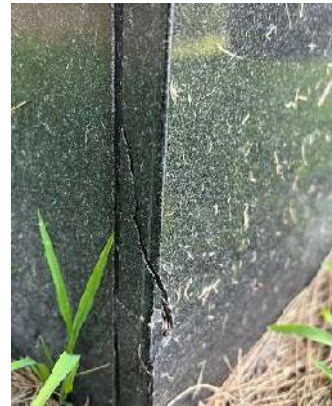
Fig 26: M5 crack and loss northeast edge
