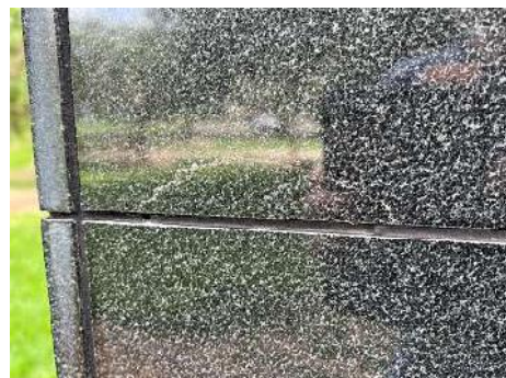
Fig 23: M4 north showing arc shaped crack and grey unpolished edge
