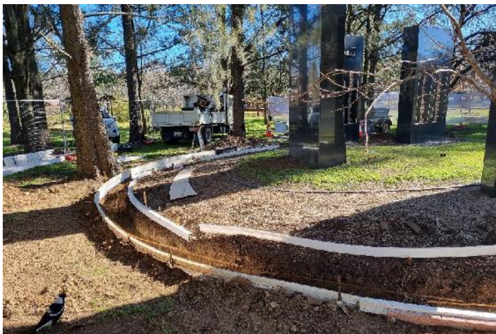
Figure 41. Photo taken during the modification works 13/07/2023 (McCann, 2023)
