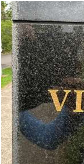
Fig 17: M2 grey area at edge loss of polished surface
