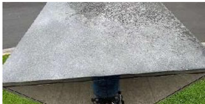
Fig 13: M1 top showing loss of polished surface
